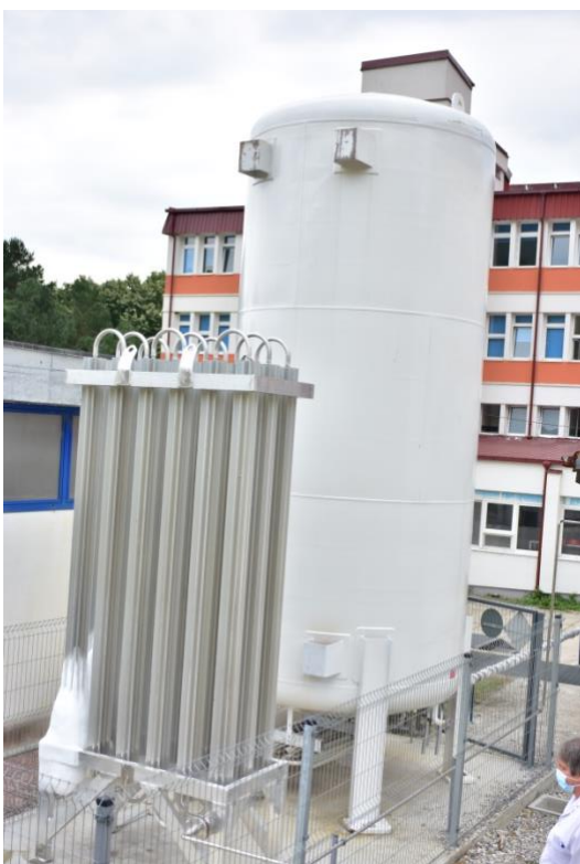
Cryo-tanku 10 ton, SP Pejë
